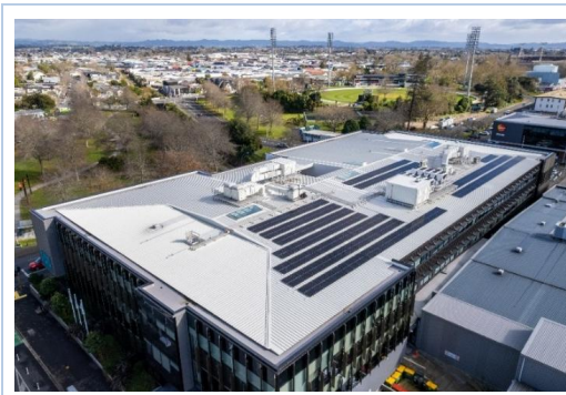
Solar panels on WRC’s main office in Hamilton
