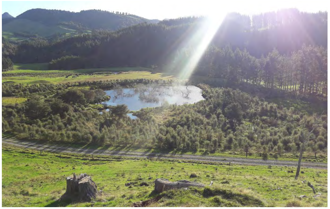
Top - retention dam. Bottom - sediment pond.
