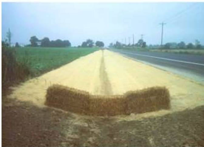
Swale construction showing erosion protection until vegetation has become established
