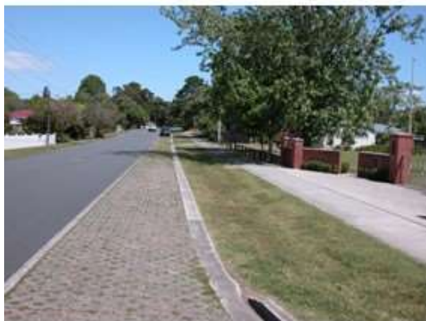
Residential Street with gobi block parking, no kerb and drainage by swale
