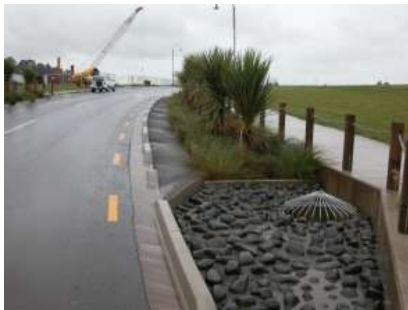
Bioretention adjacent to a road can be an attractive amenity to the overall site
