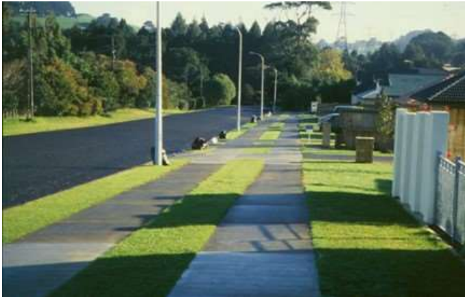
Dual pathway on one side of a street (in Auckland), increasing site imperviousness
