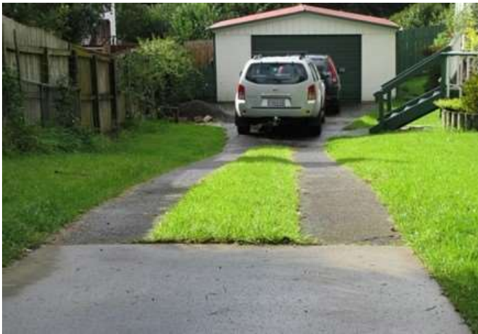
Twin concrete strip driveway reducing driveway imperviousness
