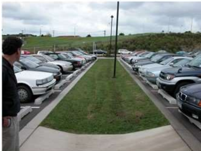
Swale with grass mowed too short and causing sediment discharge
