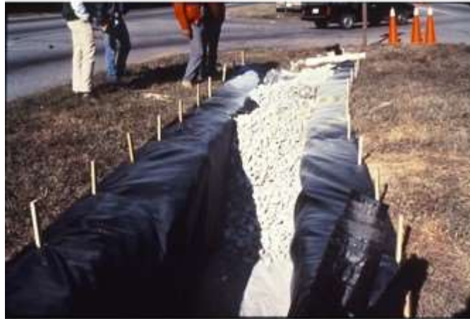
Infiltration trench backfilled with stone
