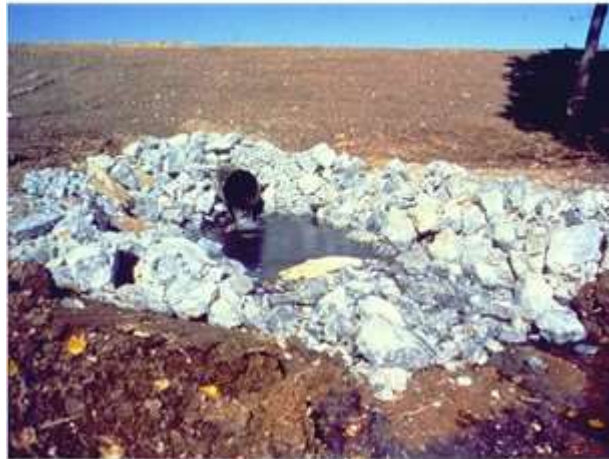
Riprap velocity dissipation at pipe outfall
