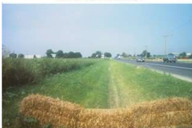
Swale with vegetative stabilisation following construction completion
