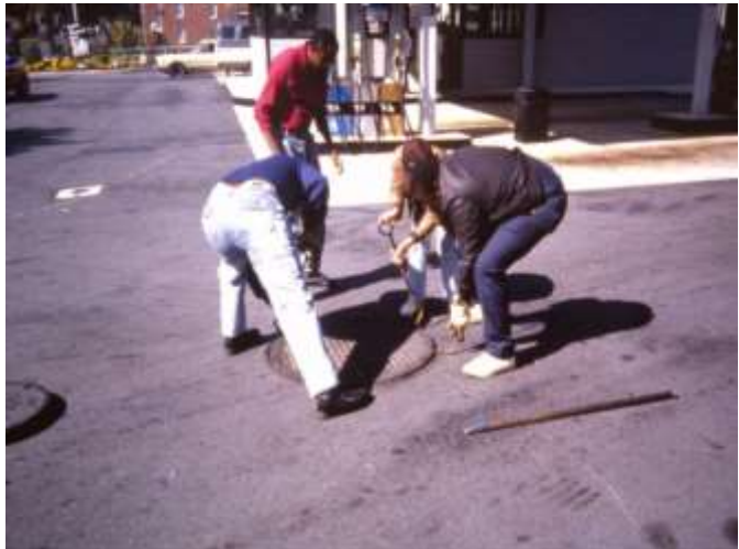
Care should be taken when removing manhole covers
