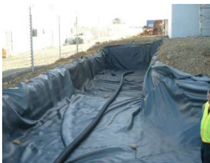
Bioretention device - lining around garden and perforated underdrain prior to backfilling
