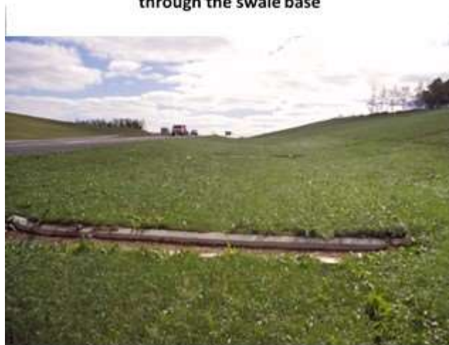
Level spreader installed to ensure dispersed flow through the swale base
