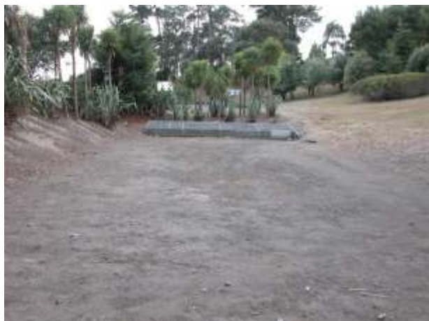
Sand filtration device at a petrol station, recently maintained
