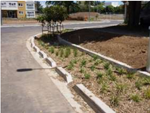
Prematurely clogged rain garden from un-stabilised adjacent areas
