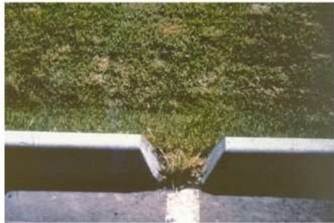
Example of a Kerb Cut
