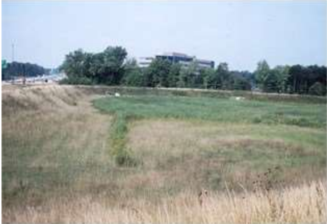
Retrofit of a dry pond with a small weir to create a wetland
