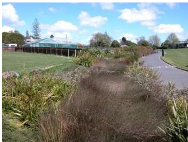
Swale using Oioi grass reduces maintenance and can be an attractive amenity
