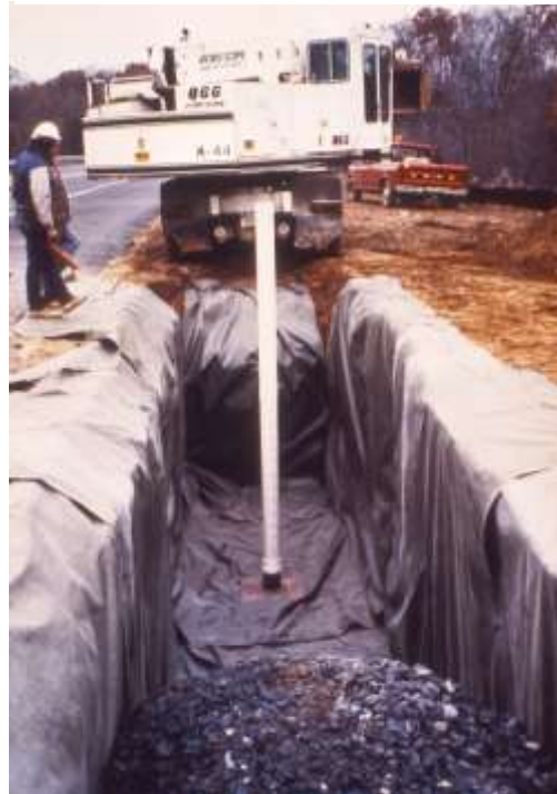
Infiltration trench - footplate and observation well
