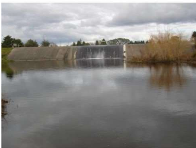
Lake Moana-nui outfall spillway
