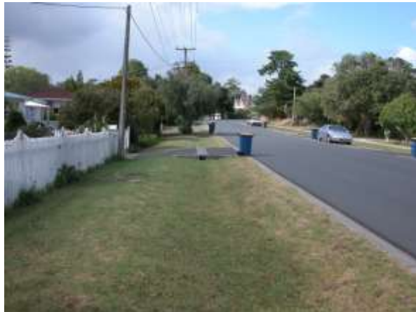
Swale treating road runoff
