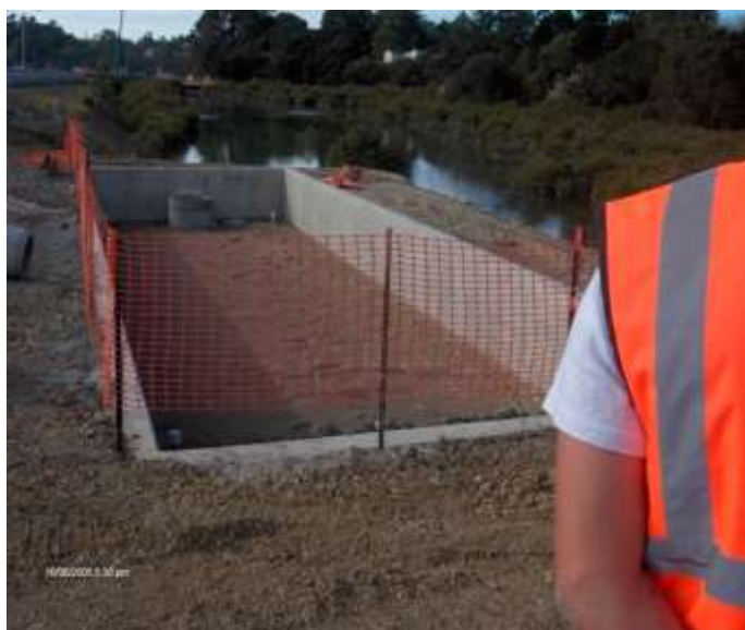
Sand filter under construction
