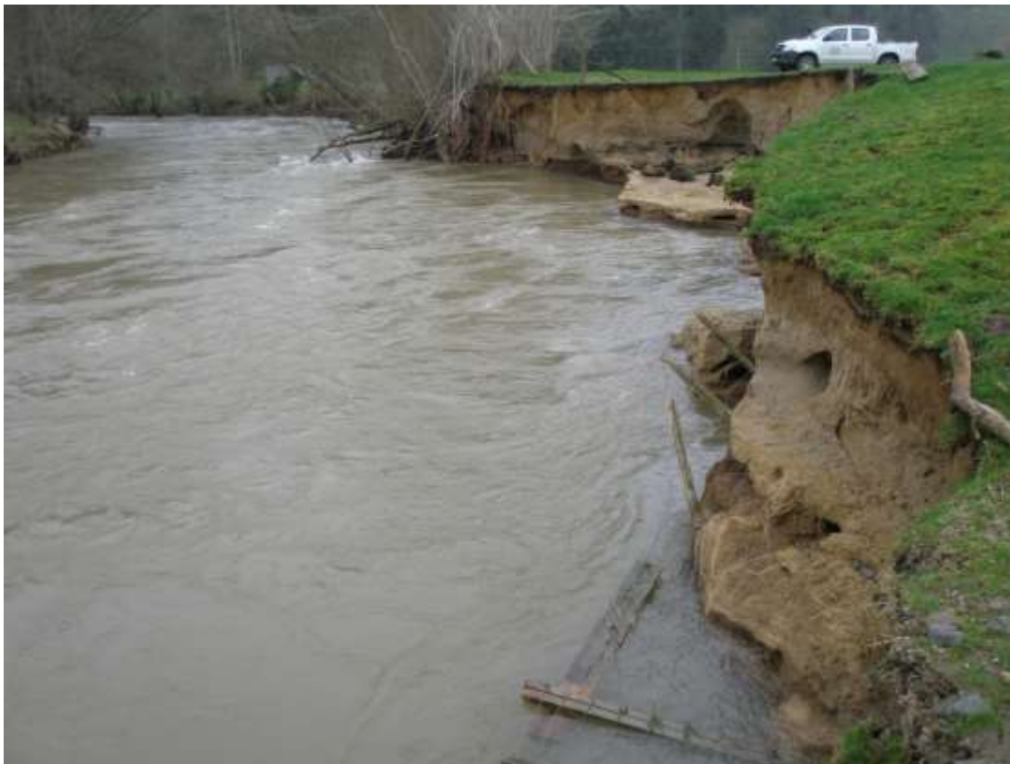
Examples of major bank erosion and instability along the Waipā River – Toa's bridge to Ōtorohanga.
