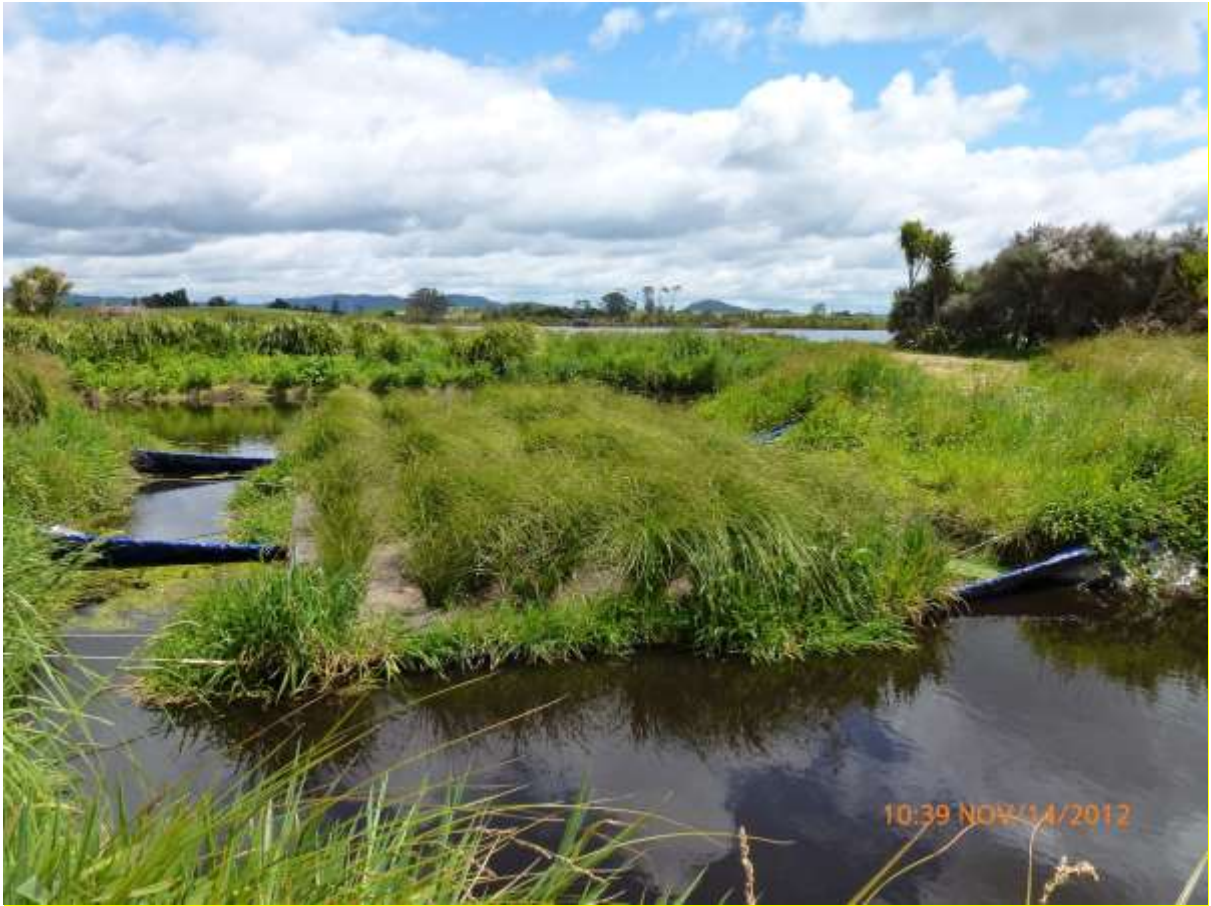
A floating wetland within one of the constructed treatment systems at Lake Kaituna.
