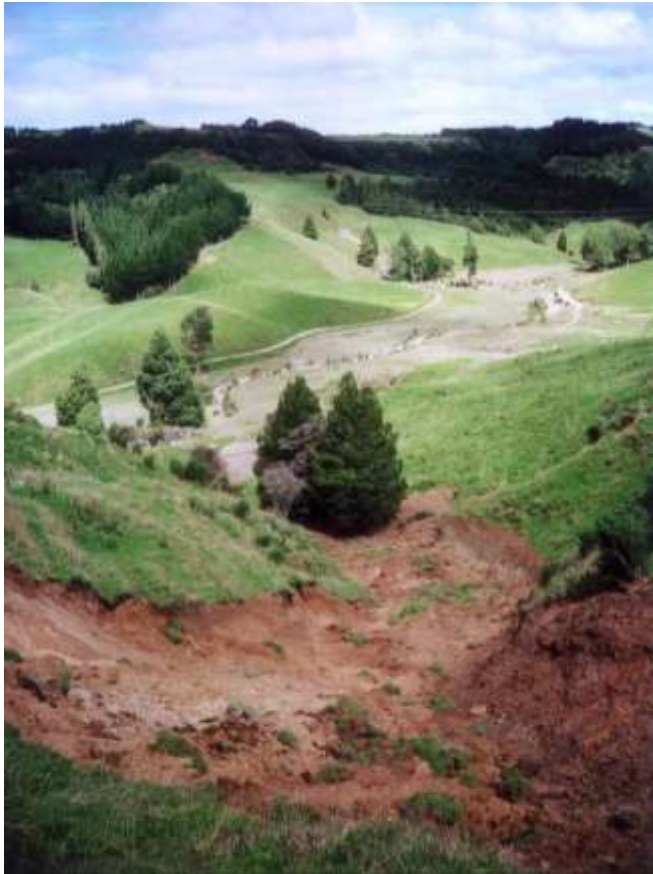
A land slip above a Waitomo stream with soil conservation afforestation in the background.
