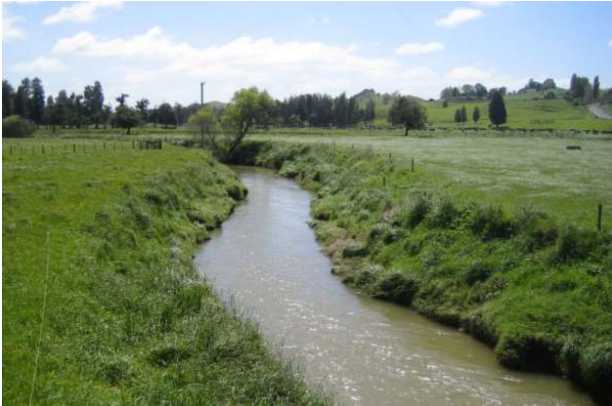
Mangapū River showing devegetated banks and lack of adequate setback.
