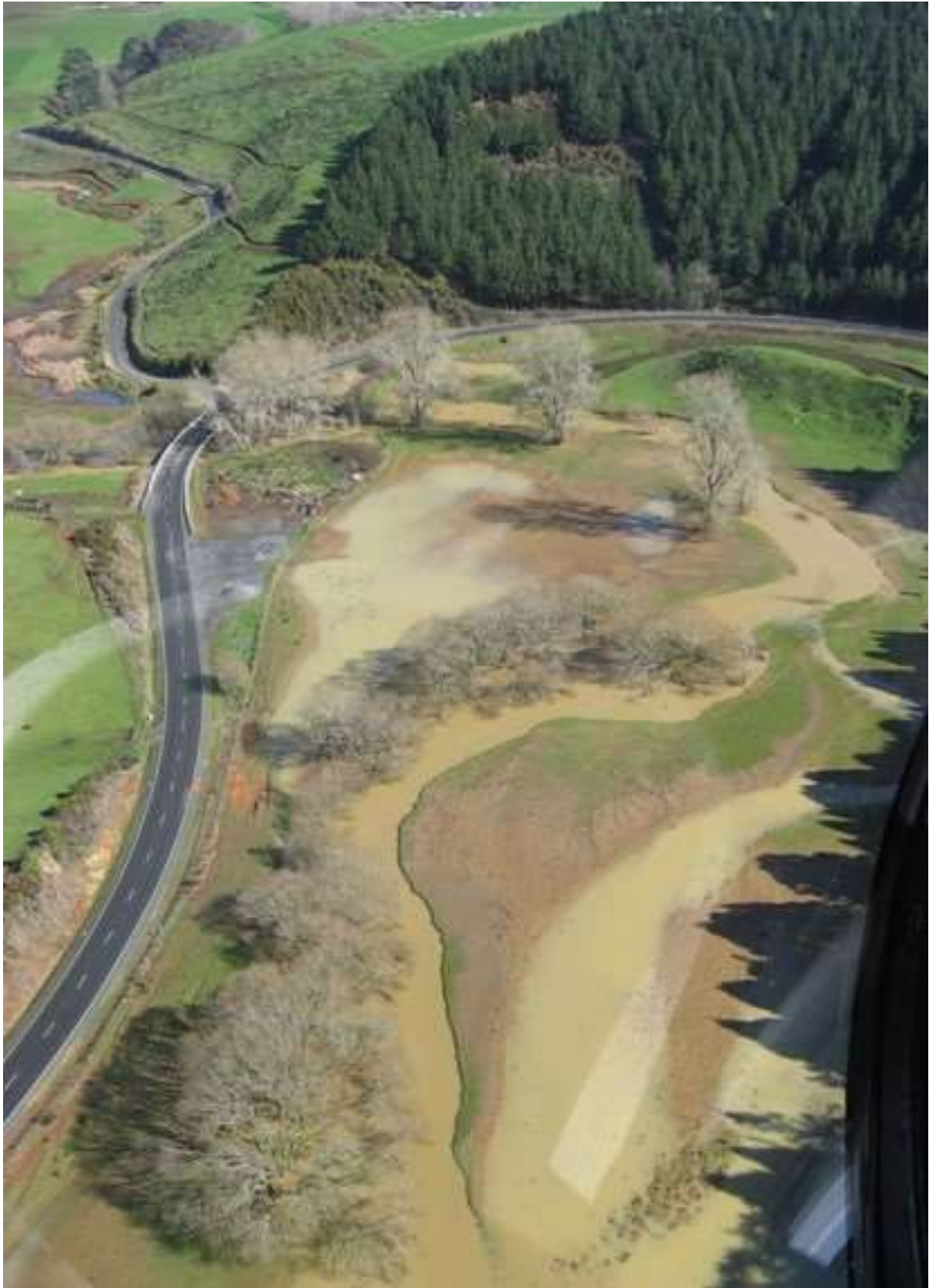
Resulting downstream sedimentation following a large weather event in the Moakurarua catchment.
