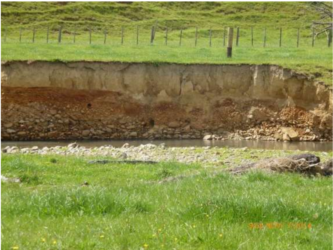
Examples of erosion along the Mangatea Stream.
