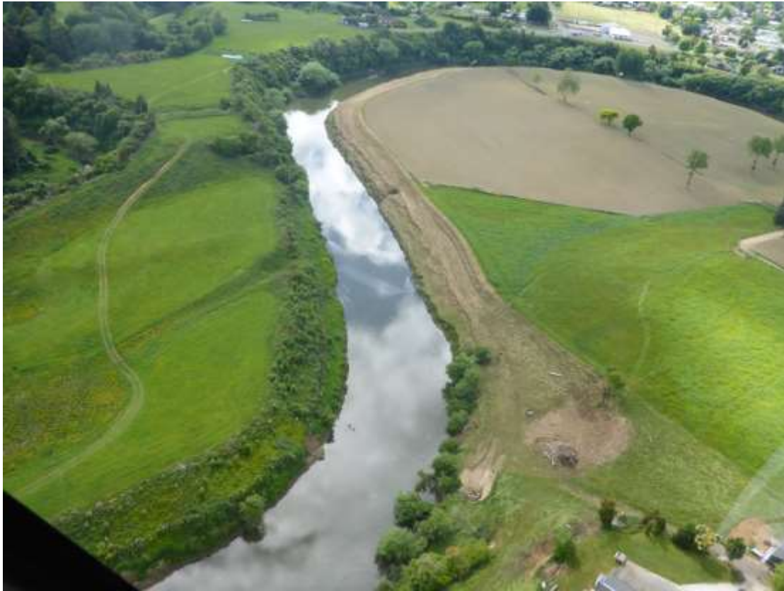
Waipā River erosion prone banks.
