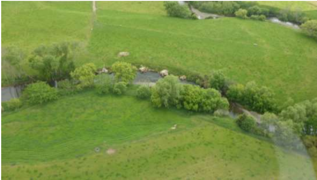
Examples of rock and vegetation erosion protection structures (as proposed as part of this project).
