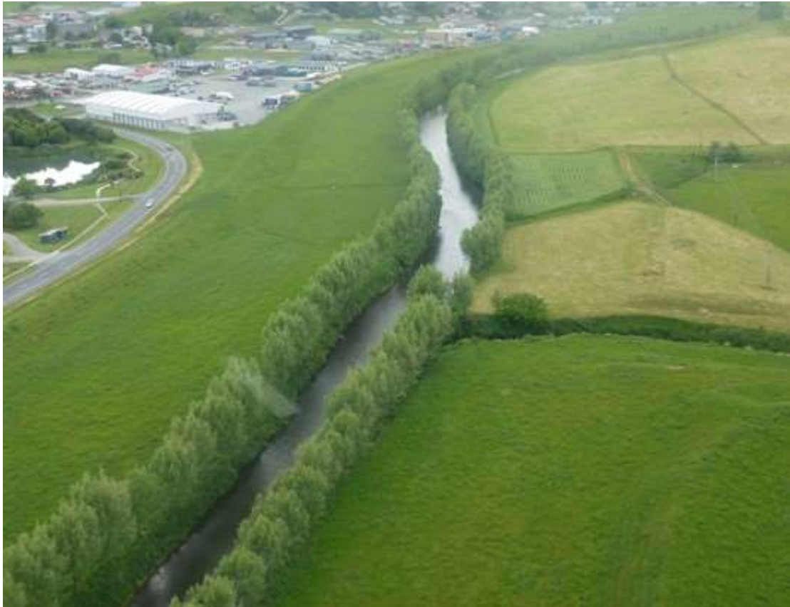
The reach of the Waipā River where work is proposed.
