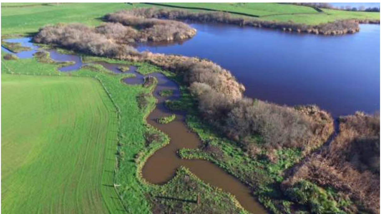
Constructed treatment system on the main inflow into Rotomanuka South (2016). (Photo: Department of Conservation)
