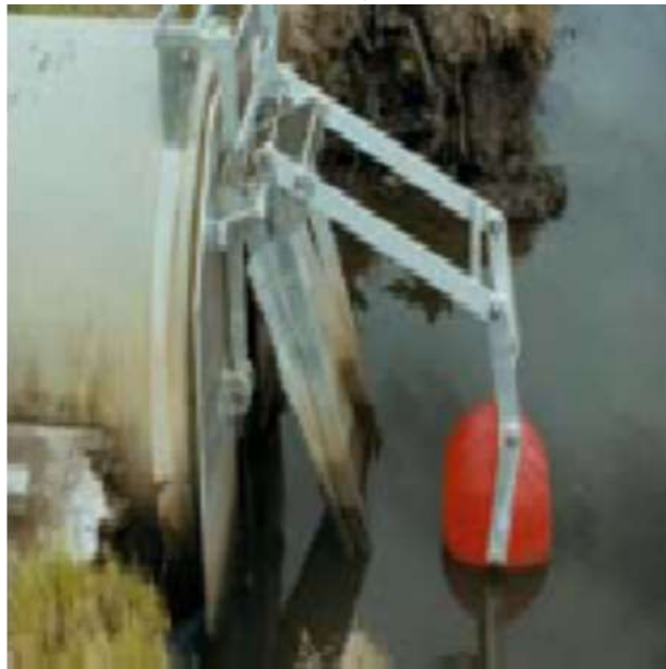
Figure 4: Example of a fish friendly floodgate. In this example, the float and lever arrangement allow a portion of the gate to remain open at levels below a pre-set maximum thus allowing unhindered upstream (and downstream) fish passage during periods of low flows.
