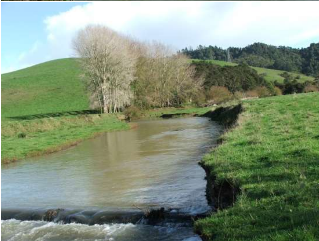
Erosion and unfenced banks along the Mangatawhiri Stream.
