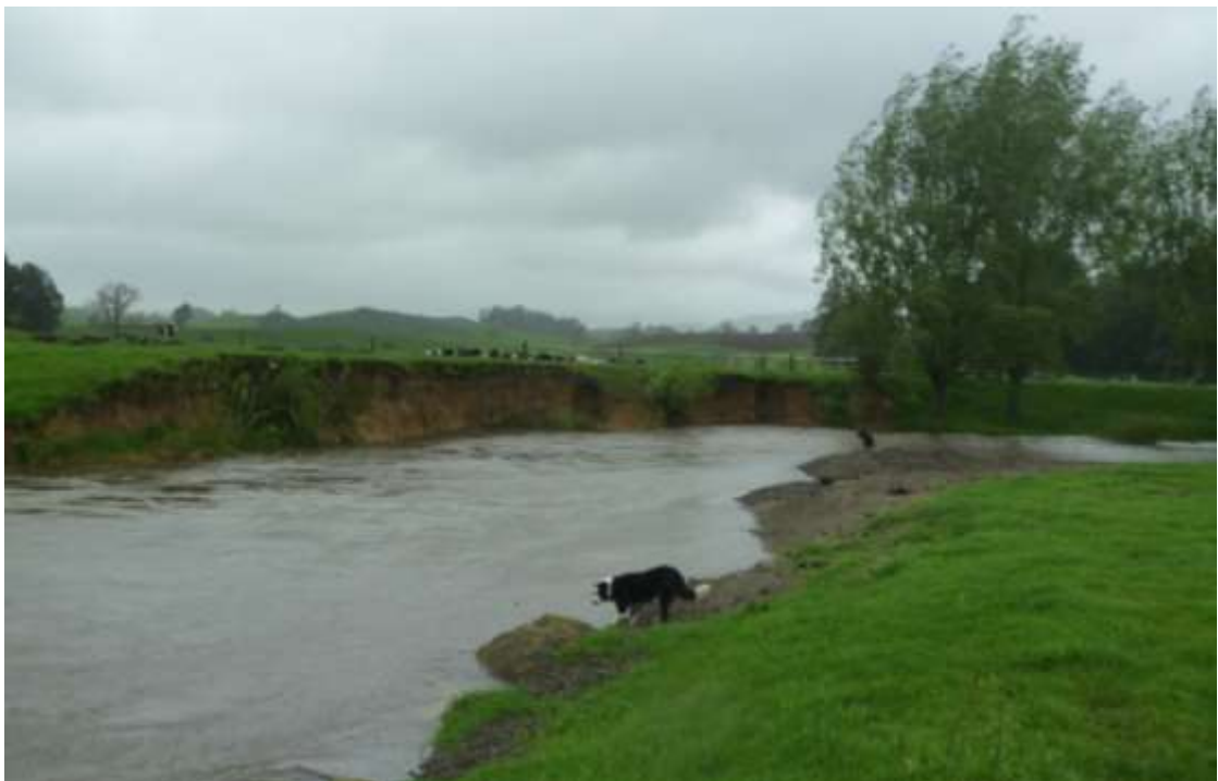
Examples of large scale bank erosion along the Mangatutu River.
