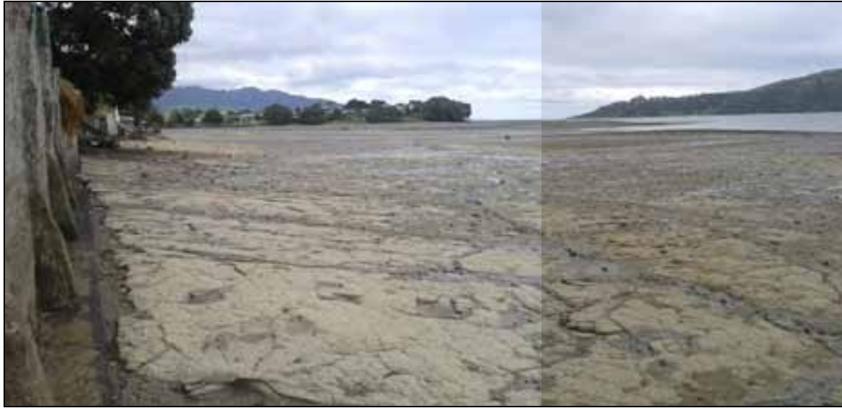
Figure 54: An armoured corner of Cox Bay showing varying styles of armouring and the natural coastal edge of the far side of the bay. Seagrass beds are visible in the middle ground and on the distant flats.
