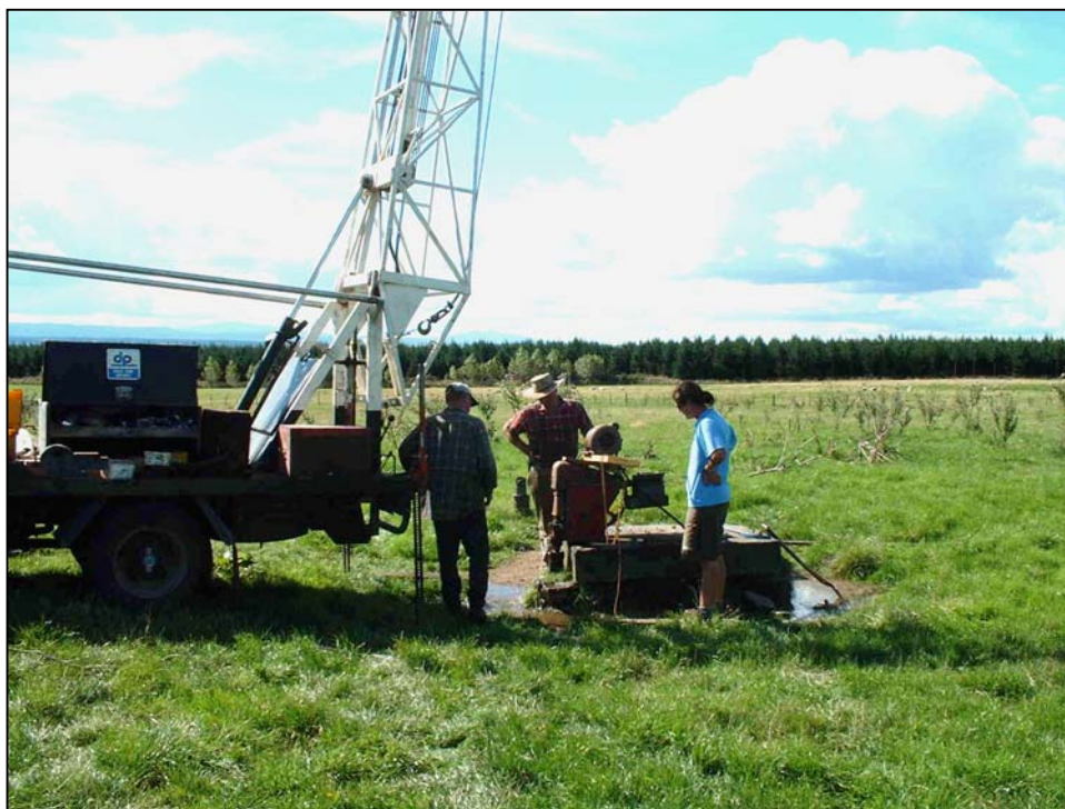
Plate 3: Lifting rig providing access to site 72.397
