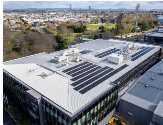
Solar panels on WRC's main office in Hamilton
