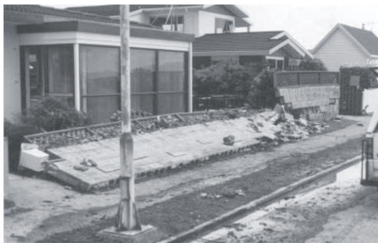
Figure 15: During cyclone Drena, wave flooding across the road caused considerable damage to property in the Thames area.
